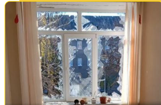
Primary Health and Sanitary Care Center" of Toretsk City
